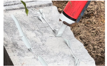
Apply QUIKRETE® Construction adhesive.
