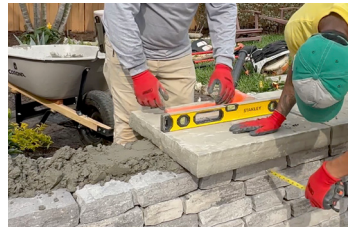
Mortar in a natural stone seat.
