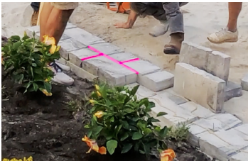
Place the next course, making sure to stagger the bond lines. Ensure level and repeat to preferred height.
